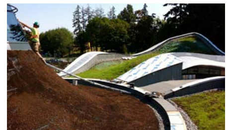
Shortly before completion of the roof surfaces.
